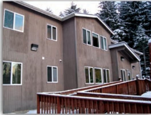
Aurora's Watch housing facility
